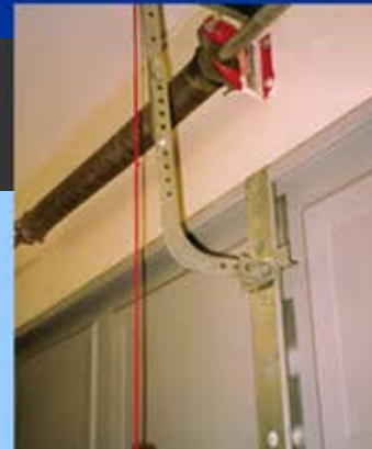
MANUAL RELEASE AND COUNTERBALANCE SPRING
